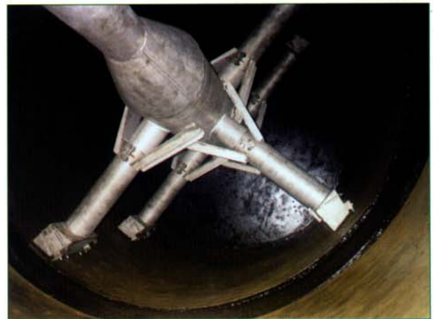
Detail of suction pipes and suction shaft of the FILTROMAX TF filter, flow 10\text{ m}^3/\text{s}
