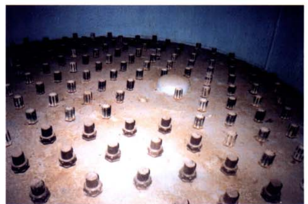
Fitting of sand filter PFZ
