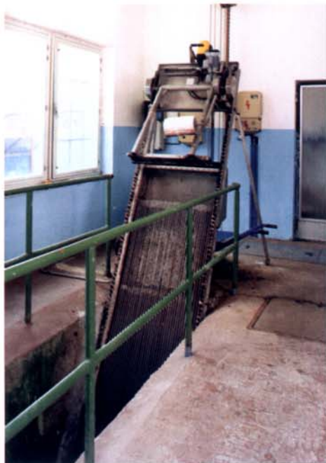
Truck screen in WWTP, CR
