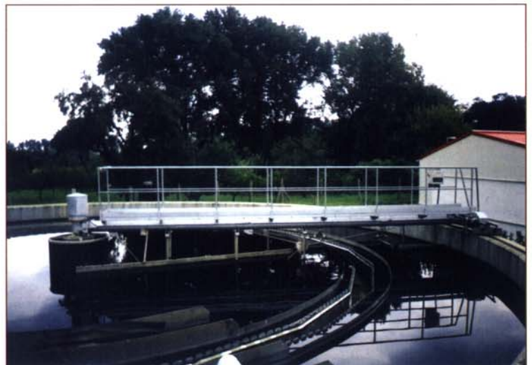
Secondary sedimentation tank
