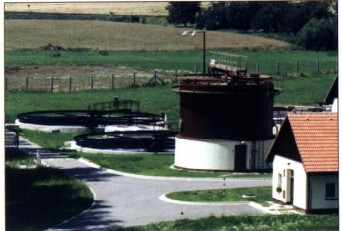
Sedimentation and thickening tanks at WWTP, CR
