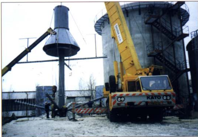
Erection of ZN 12/12 for kaolin
